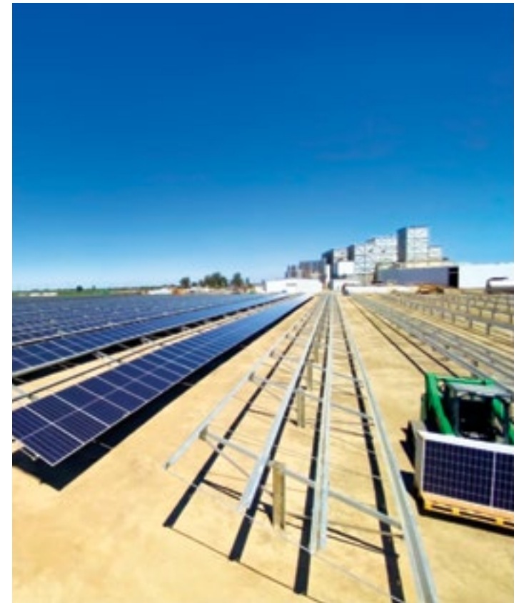
In 2021, we began work on a 10-megawatt solar project on 13 acres at one of our facilities in Lemoore, Calif. The electricity will contribute approximately 10% of the plant's annual energy needs.
